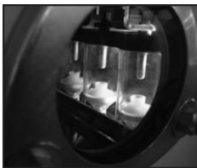
◀ Load break switch visible break.
