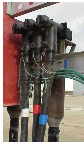
15/25kV dead-end joint in a substation application.
