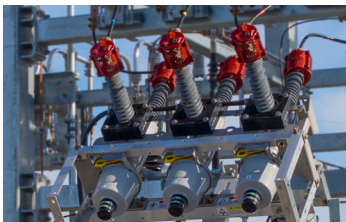
Viper-ST with one set of external CTs. A second set of CTs can be provided on the other side.
