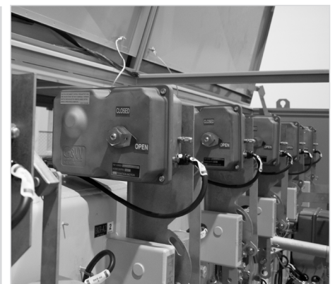
Motor actuators can be added for remote operation.
