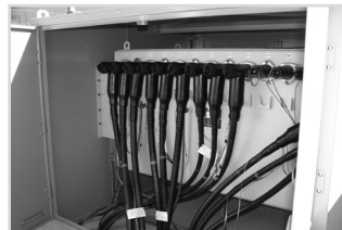
Cable entrances are located on the back of the switch.
