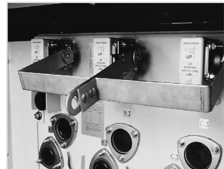
Three phase interrupter operating handle
