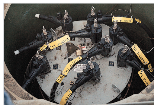
RP style switches can be floor, wall or frame mounted in any altitude.
