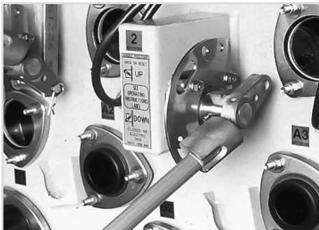
Fault interrupter operating handle
