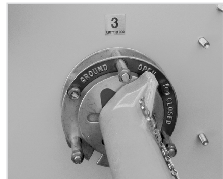
Load break multi-position switch operator
