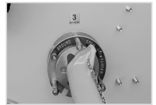
Load break multi-position switch operator
