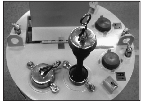
Canister fuses incorporate a provision for hookstick removal and replacement.
