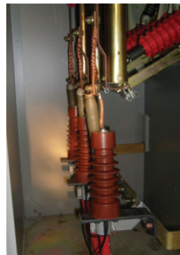
24kV Voltage Sensor installed in switchgear application
