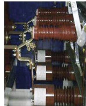
Voltage Sensor (VS-24-I – top) & Current Voltage Sensor (CVS-24-I – bottom) installed in switchgear application
