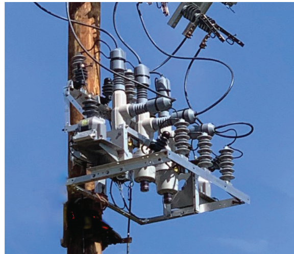
Protection and Metering: Overhead platforms install on G&W Electric Viper®-ST Recloser (VS-27-0)
