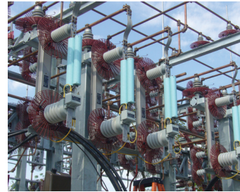
CLiP installed in a generating station at a large southeastern university
